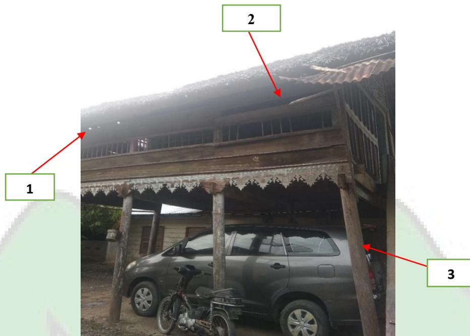
Gambar 3. 8 Keadaan Rumah 1. Atap bocor, 2. Dinding bolong, 3. Tiang miring
