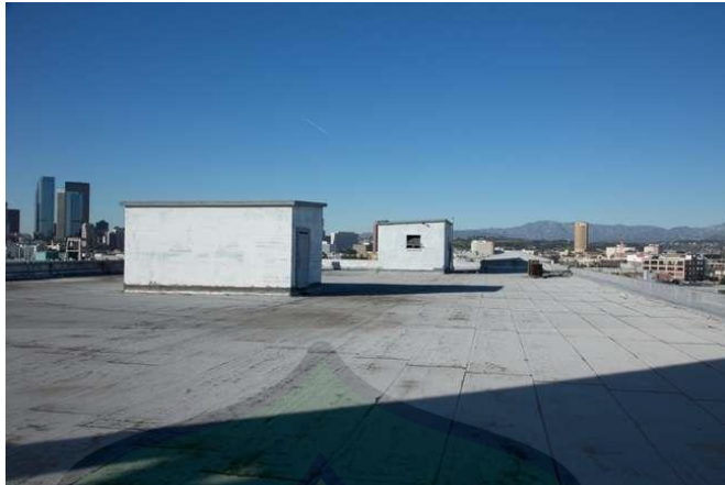
Gambar 4.69 : atap dak beton
