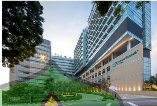
Gambar 2. 12 Tampak Bawah Mount Elizabeth Hospital (Sumber: mountelizabeth.com.sg)
