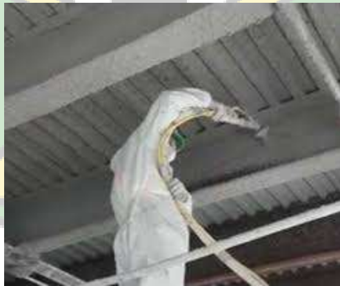
Gambar 5. 40 Proses Fire Proofing
