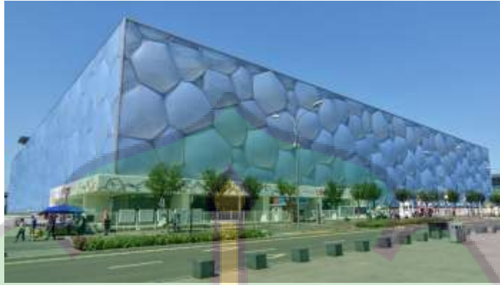
Gambar 3. 14 Water Cube Aquatic Center
