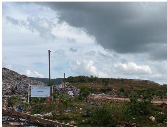
Gambar 2. 1 Controlled Landfill TPA Regional Blang Bintang
