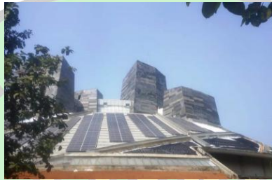
Gambar 3 4 Solar Panel Universitas Indonesia
