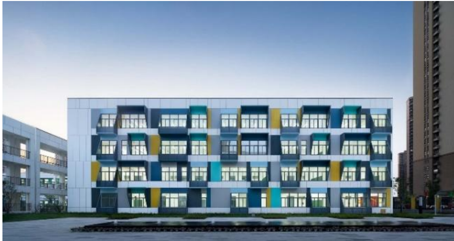
Gambar 3. 1. Fasad Bangunan School Nanjing , China
