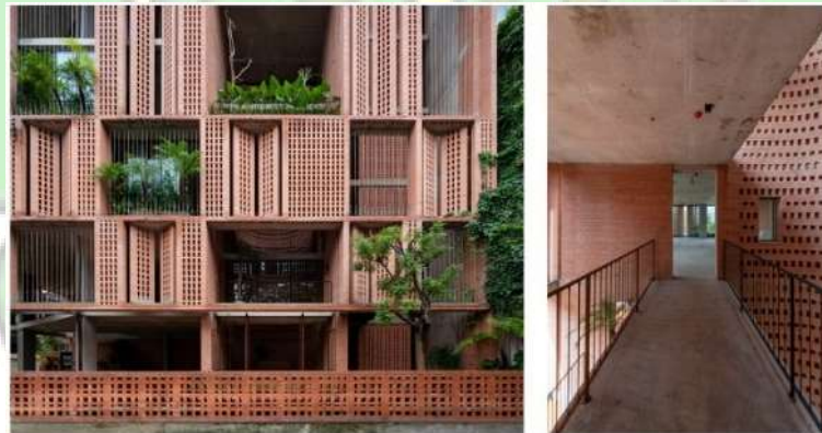
Gambar 3. 8 Fasad & Void Premier Office
