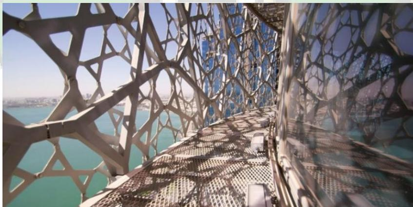
Gambar 5.8 : GRC (Glassfibre Reinforced Concrete)
