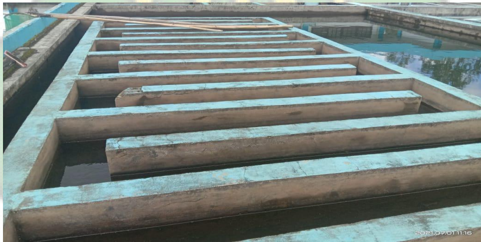
Gambar 4.6. Bak Flokulasi ( buffer channel )
