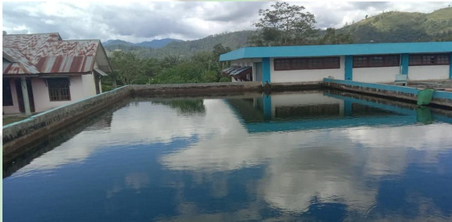
Gambar 4.4Bak Prasedimentasi
