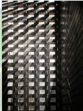
Gambar 5.7 Breeze Block (Roster Beton)
