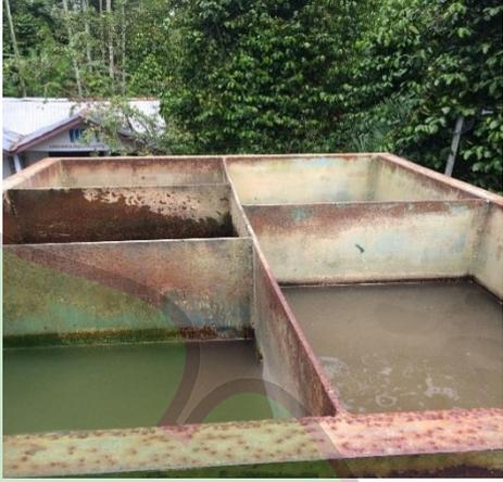
A photograph of a sedimentation tank at the IPA PDAM Tirta Krueng Meureudu. The tank is divided into sections and contains a layer of sediment at the bottom. |
