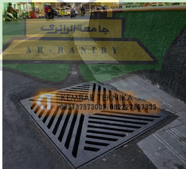
Gambar 4.18 Grill Cover drainase
