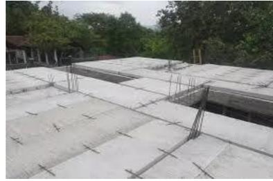
**Gambar 5.32** Atap dak beton
