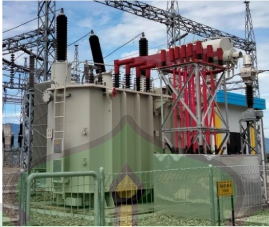
Gambar 3.6 Transformator Daya 60 MVA UNINDO
