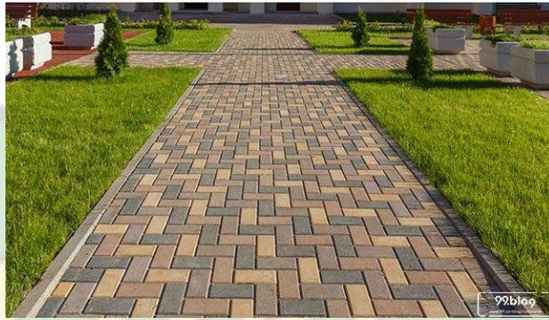
Gambar 5.17 Paving block
