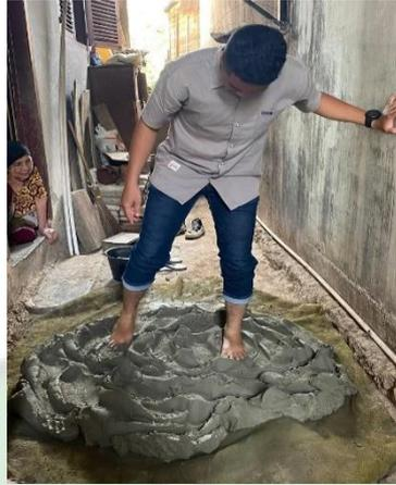
Gambar 3.17 Proses Injak-Injak Tanah
