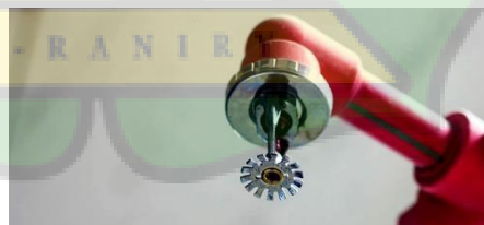
Gambar 4.51 sprinkler Sumber: firecek
