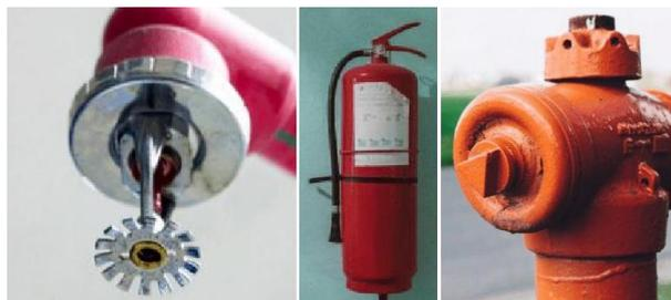
**Gambar 5.26** Sprinkler, Fire Extinguisher, Hydrant
