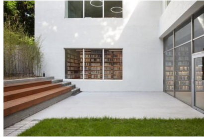
Gambar 2.34. Gambar perpustakaan renovasion cultural geumcheon (Smber: arch daily 2021)
