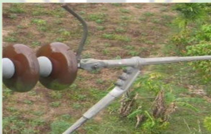
Gambar 2.6 Gambar jumper joint
