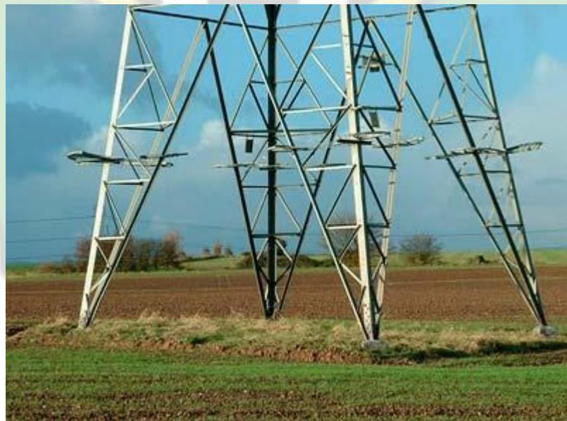
Gambar 2.17 Anti *Climbing Device* (ACD)
