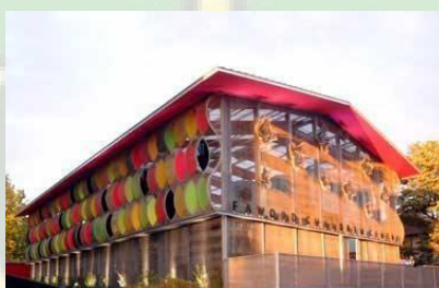
Gambar 3.1 Eksterior Bangunan Fawood Children's Center London, UK Sumber: https://arcSPACE.com .
