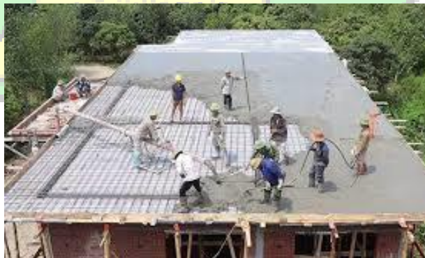
Gambar 5.16 Atap Dak Beton
