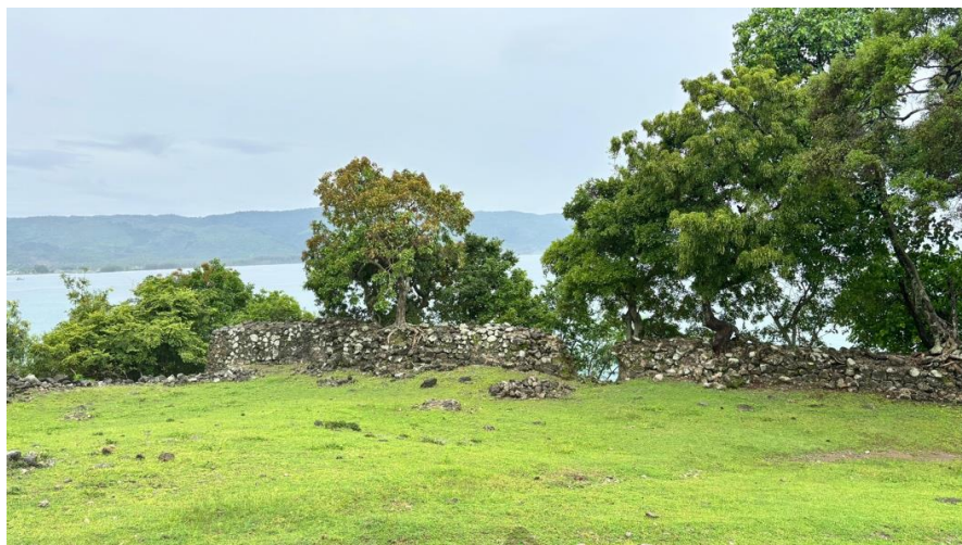
Figure 1. Condition of the back of Inong Bale Fort
