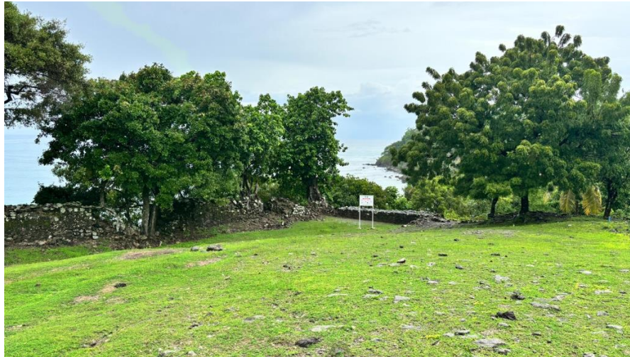
Figure 2. Condition of the side of Inong Bale Fort
