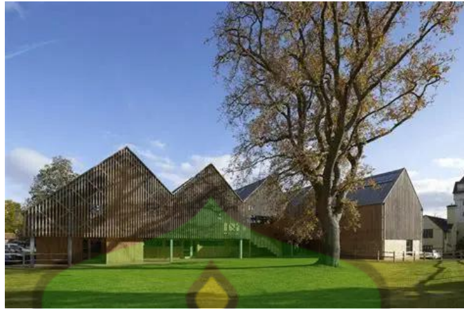
Gambar 3. 1 Bangunan Badales School Art and Design (Sumber : archdaily.com, 2025)
