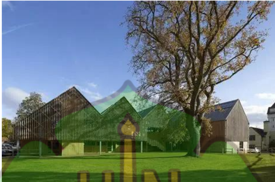
Gambar 2. 23 Bangunan Badales School Art and Design (Sumber : archdaily.com, 2025)
