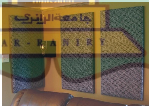
Gambar 4. 12 Panel Akustik Fabric + Rockwool
