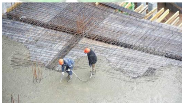
Gambar 4.39 Atap dak beton
