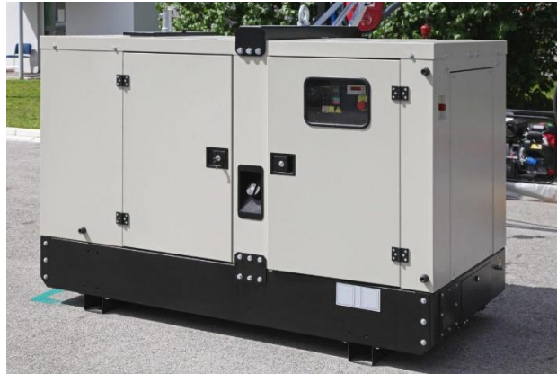
Gambar 4.42 Generator cadangan (genset)
