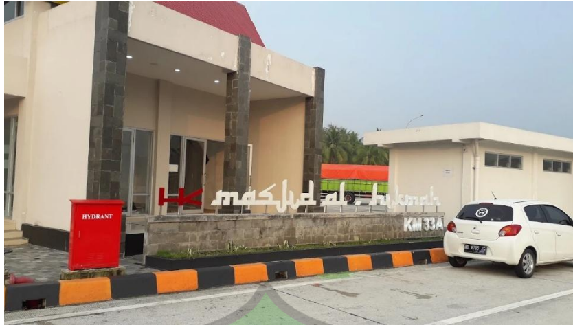
Gambar 2.19 Rest Area KM 33 A/B Tol Bakauheni-Terbanggi Besar (Sumber: https://hkinfrastruktur.com )
