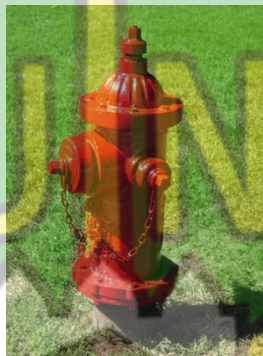
Gambar 5.25 Hydrant (Sumber: Pinterest)
