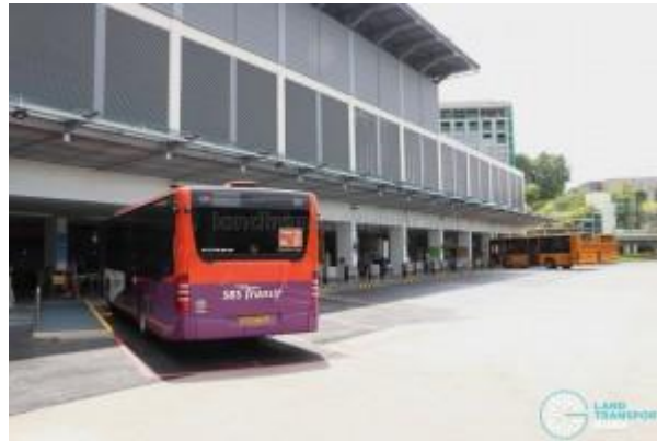
Gambar 3. 5 Beach Station Bus Terminal – Parking Lots Sumber: Landtransportguru.net, 2025
