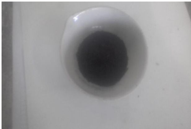
Zat Adiktif Abu Boiler
