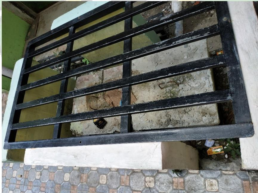
Gambar 4.4 Bak *Grease Trap*
