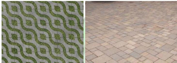
Gambar 3.28 : Material grass block dan paving block
