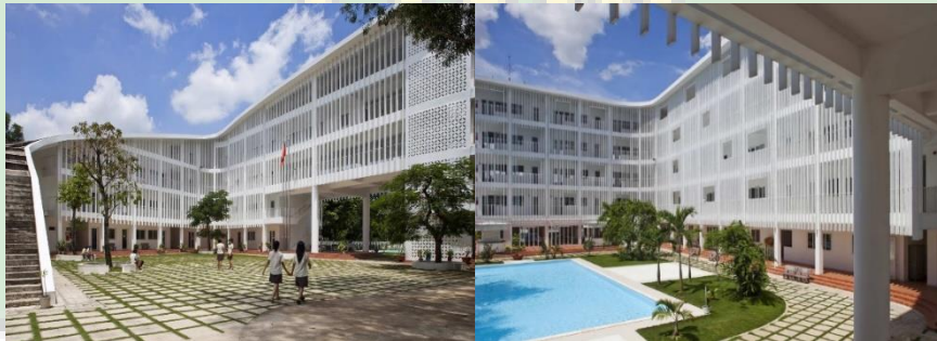
Gambar 3.29 Ruang Luar Binh Duong School Sumber: Archdaily.com (2012)
