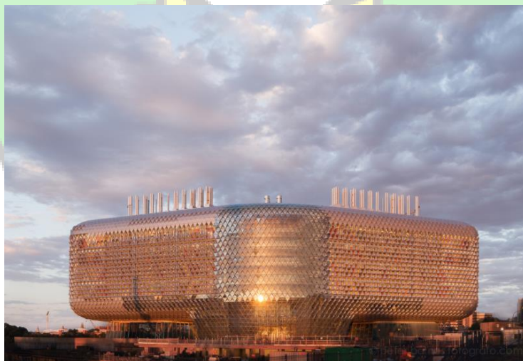
Gambar 3.13 SAHMRI Building, North Terrace, Adelaide Sumber: www.inhabitat.com
