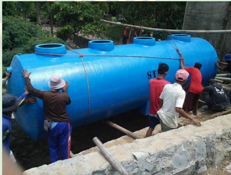
Gambar 5.15 Bio Septic Tank
