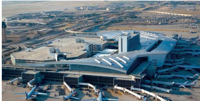
Gambar 3.4: Terminal Bandara International Dallas / Forth Worth
