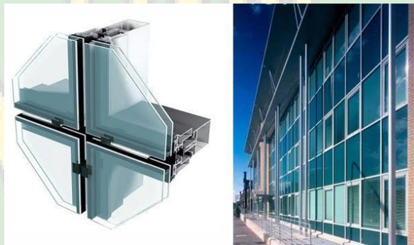
Gambar 3.1: Detail Curtain Wall
