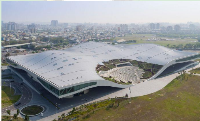
Gambar 2.88: National Kaohsiung Centre for the Arts (Sumber: https://idea.grid.id/ )
