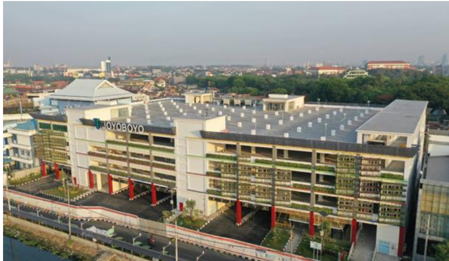
Gambar 3. 24 Green fasade terminal joyoboyo Sumber : https://dishub.surabaya.go.id
