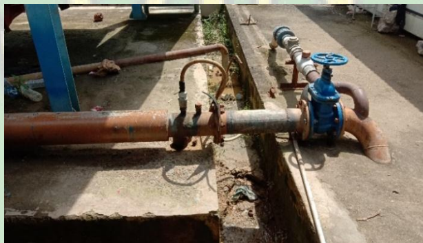
Gambar 4.7 Selang Penginjeksian Koagulan
