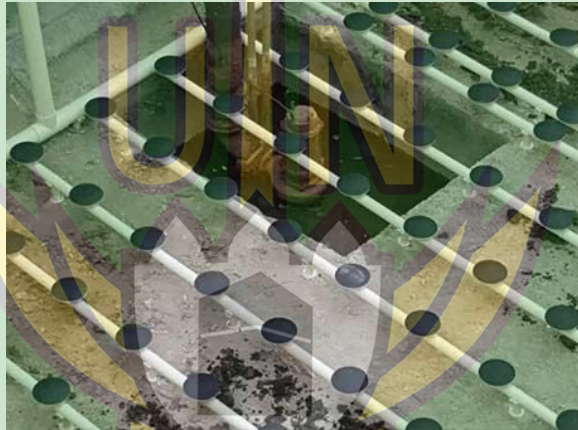
Gambar 4. 7 fine bubble tube difuser
