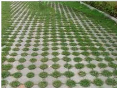
Gambar 5. 24 *Paving Block* Berpori
