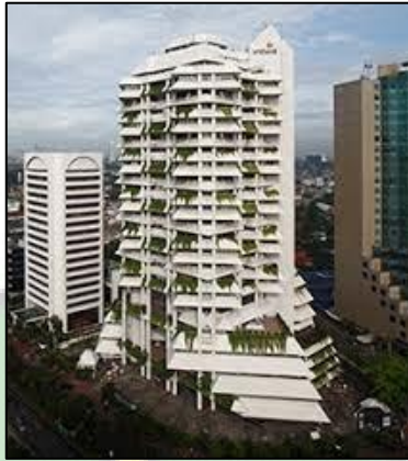
Gambar 3. 31 Gedung Wisma Dharmala Sakti
