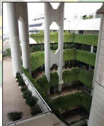
Gambar 3. 32 Interior Void Wisma Dharmala Sakti
