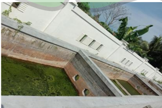
Gambar 3.8 Bak Resapan Limbah Cair UPTD RPH Lambaro
