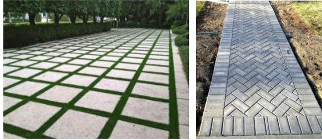
Gambar 5. 10 Grass Block Dan Paving Block
