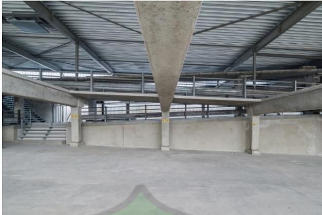
Gambar 3. 28 Struktur Balok Dan Material Bondek Di Plafon Bangunan World of Food Shopping Centre
