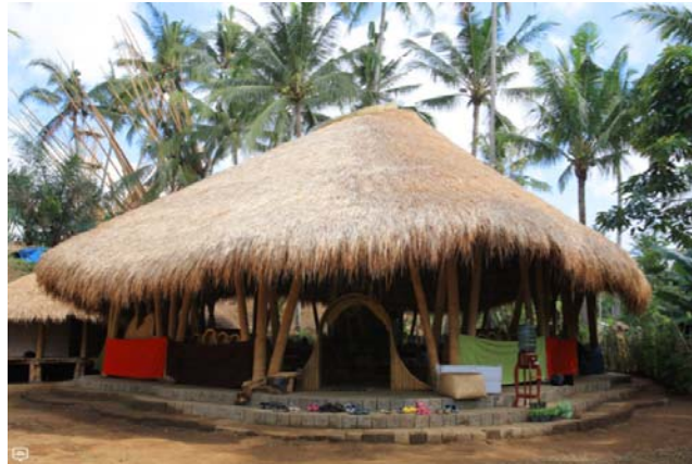
Image 3. Green School Bali building Source: IBUKU
