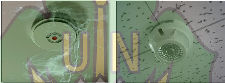
Gambar 5.36 smoke detector , heat detector . (Sumber: Sewakantor.com)
