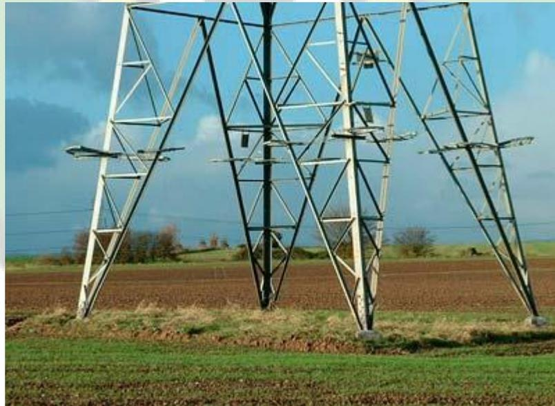
Gambar 2.17 Anti *Climbing Device* (ACD)
