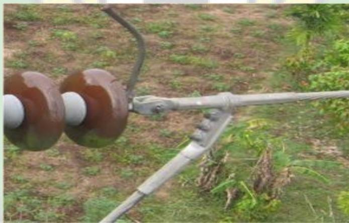
Gambar 2.6 Gambar jumper joint
