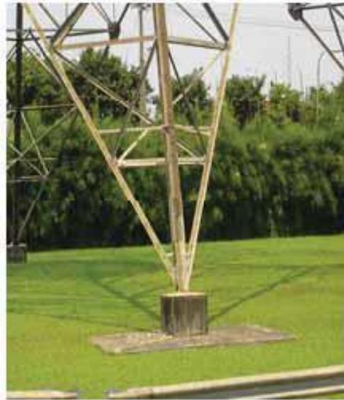
Gambar 2.13 Pondasi Tower (*lattice*) SUTET 500 kV Gresik - Krian
