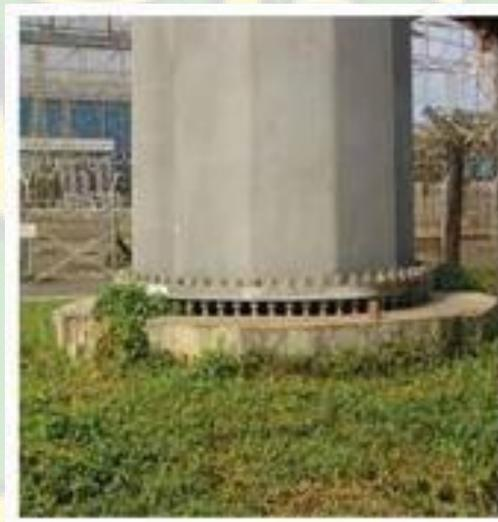
Gambar 2.14 Pondasi *Steel* 500KV *Dead End* Suralaya
