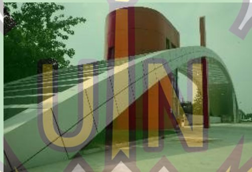
Gambar 6.6 Material Atap Aluminium Composite Panel
