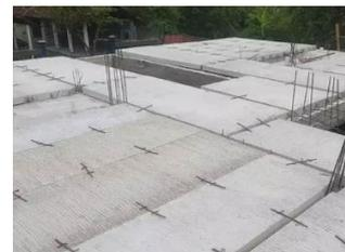
**Gambar 5.24** Atap Dak Beton
